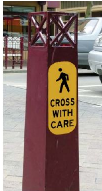
Photo 15.10 – Sign on bollard delineates edge of roadway, Palmerston North (Photo: Tim Hughes)
