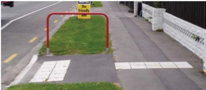
Photo 15.4 – Kerb ramp, near bus stop, SH 1, Russley Rd, Christchurch (Photo: Tim Hughes)
