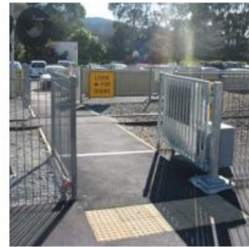
Photo 15.25 – Automatic pedestrian gate, Upper Hutt (Photo: Roy Percival)
