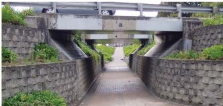
Photo 15.14 – Underpass, Pukete, Hamilton (Photo: Tim Hughes)
