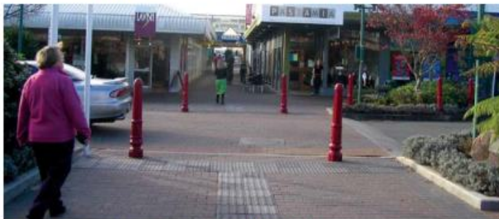
Photo 15.5 – Blended kerb crossing at platform, Taupo (Photo: Else Tutert)
