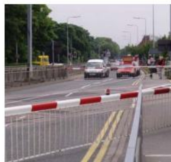
Photo 15.23 – Full automatic barriers, Hull, U.K. (Photo: Tim Hughes)
