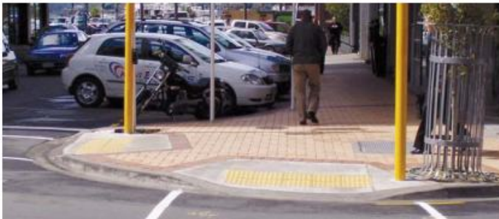
Photo 15.3 – Kerb ramp, Featherston St, Wellington (Photo: Tim Hughes)
