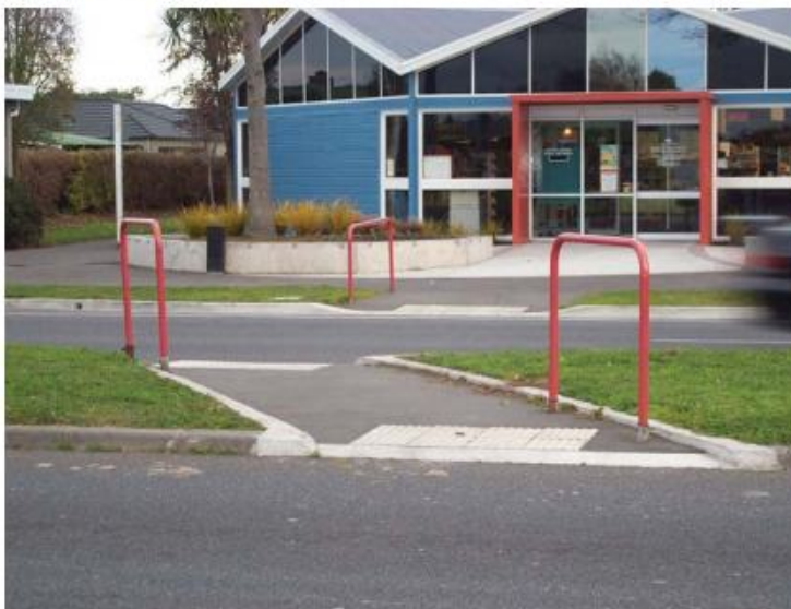
Photo 15.8 – Median with path cut through Island, SH 74 Main Nth Rd, Christchurch (Photo: Susan Cambridge)
